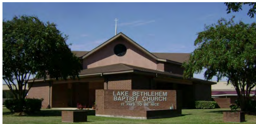
LAKE BETHLEHEM BAPTIST CHURCH 2842 DR. MARTIN LUTHER KING DRIVE SHREVEPORT, LOUISIANA
